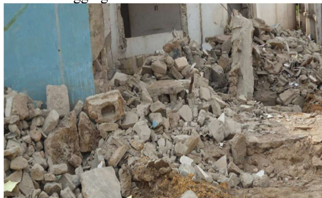
Figure 2: Demolished Wall Source of Recycled Concrete Aggregate
