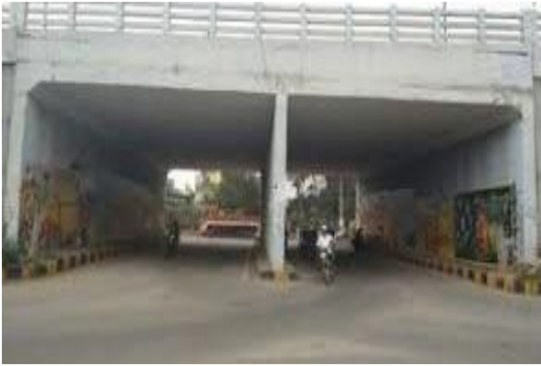
Fig 1.2 VUP & PUP type Underpass (Ref- Highway Correspondence)
